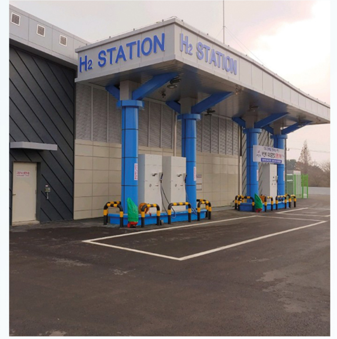
Seosan Fueling Station
