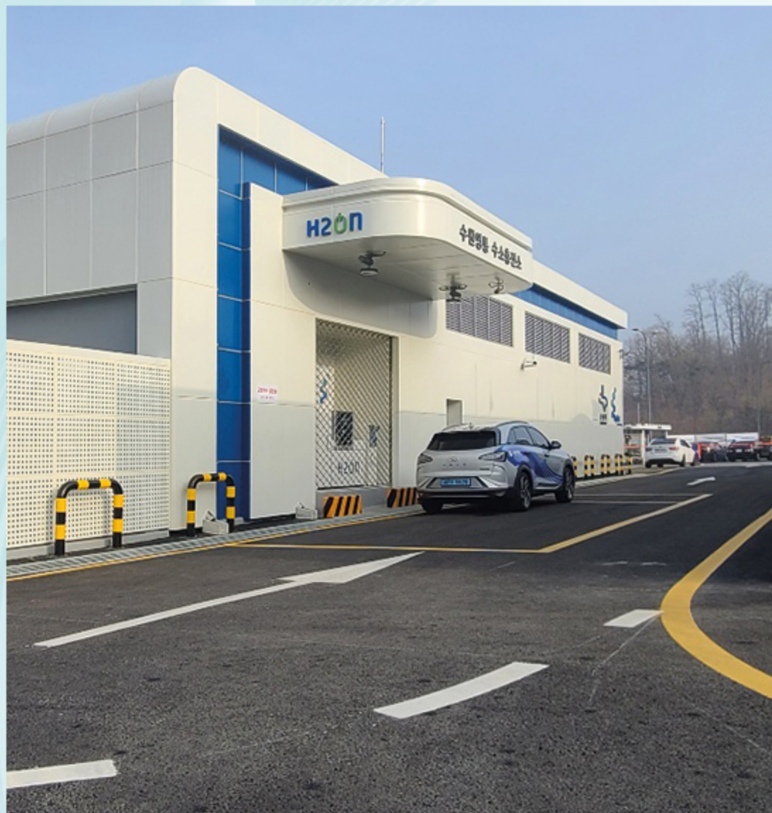
Suwon Gwanggyo Fueling Station
