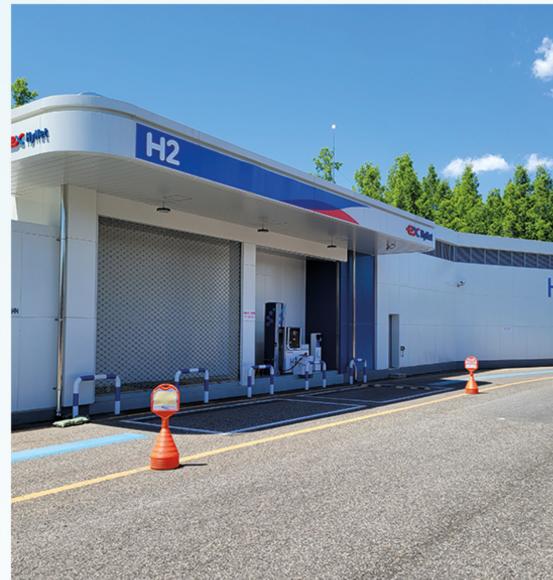
Sintanjin Fueling Station
