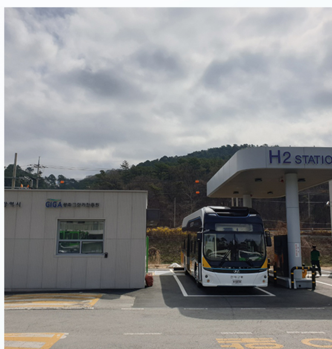
Gwangju Fueling Station
