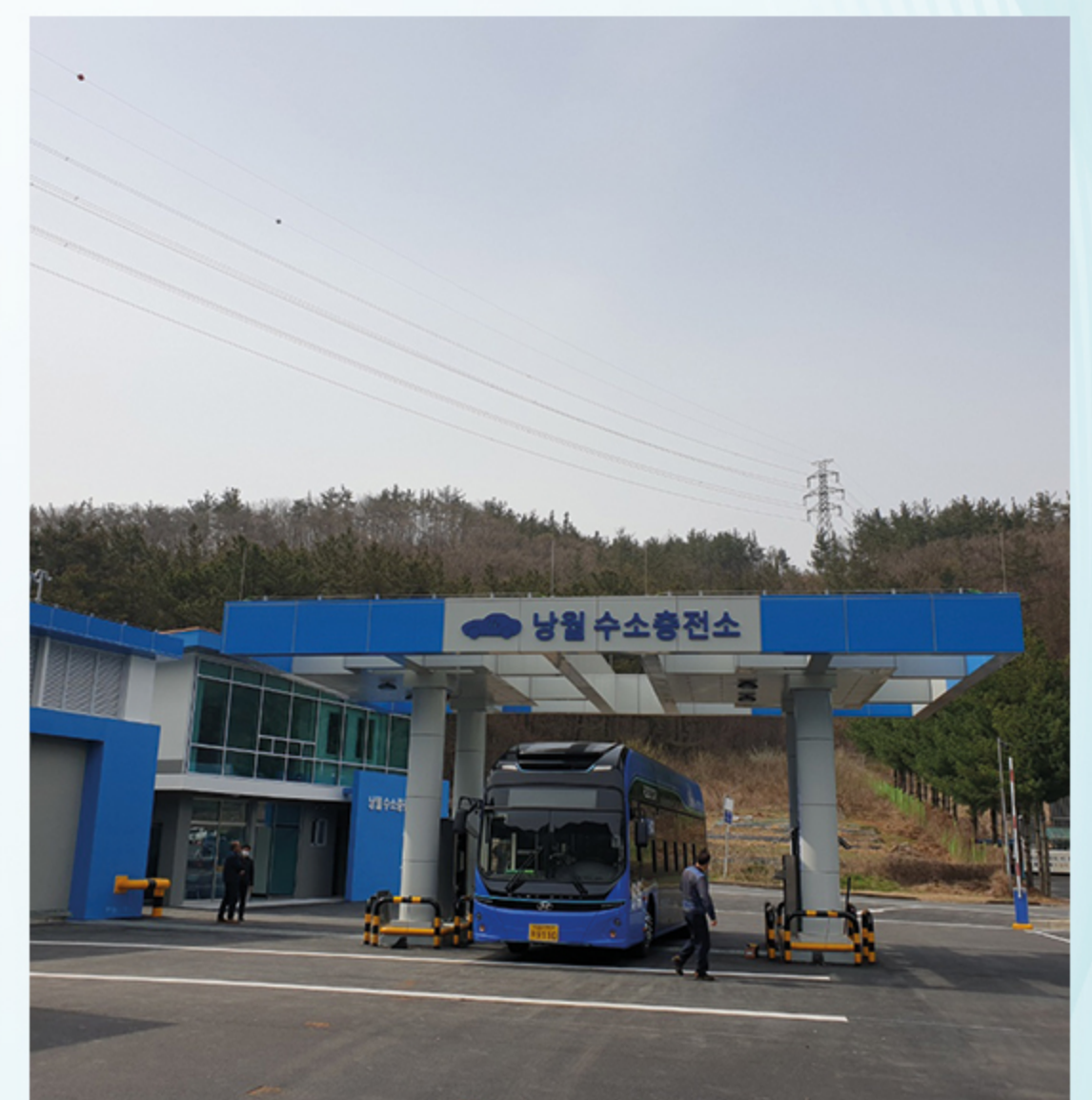
Daejeon NangWol Fueling Station
