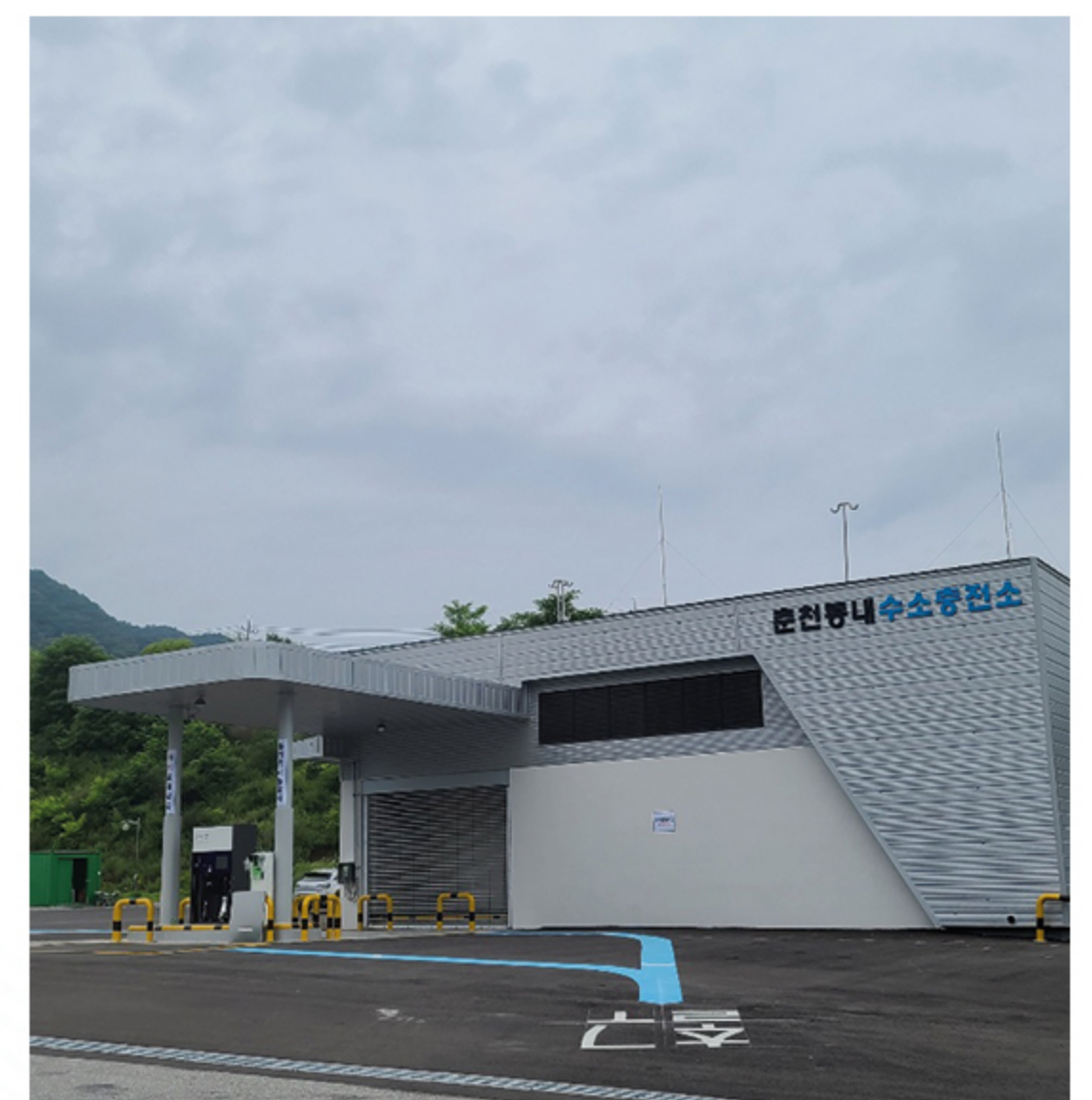
Chooncheon Fueling Station
