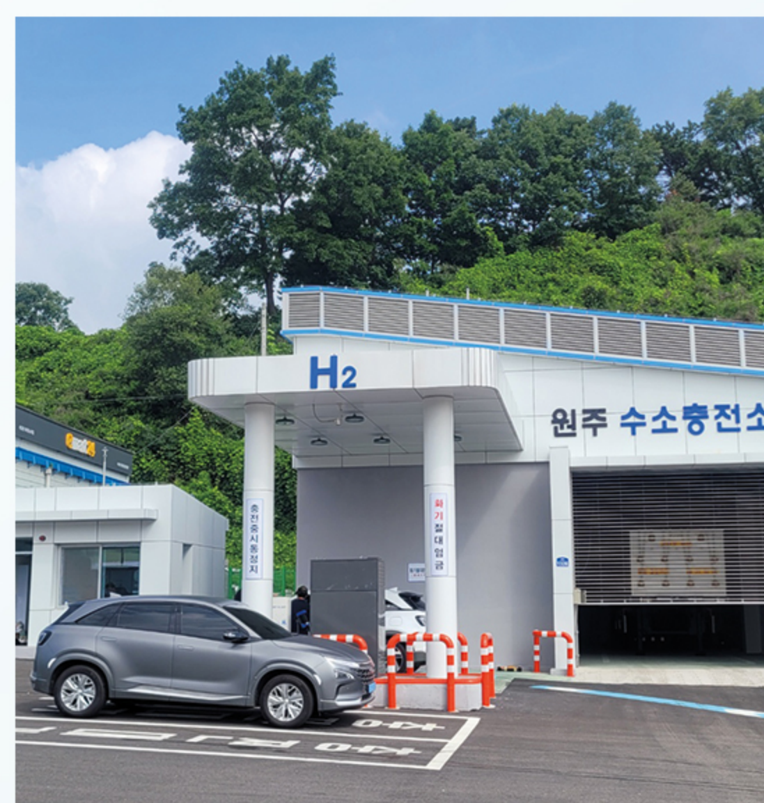
Wonju Fueling Station
