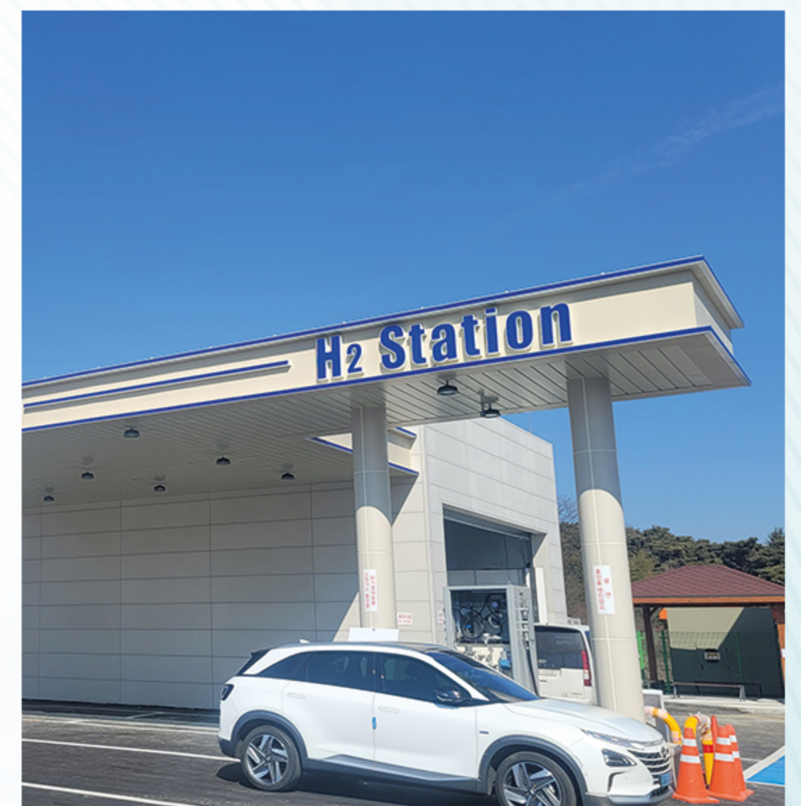
Jeonju Samcheon Fueling Station
