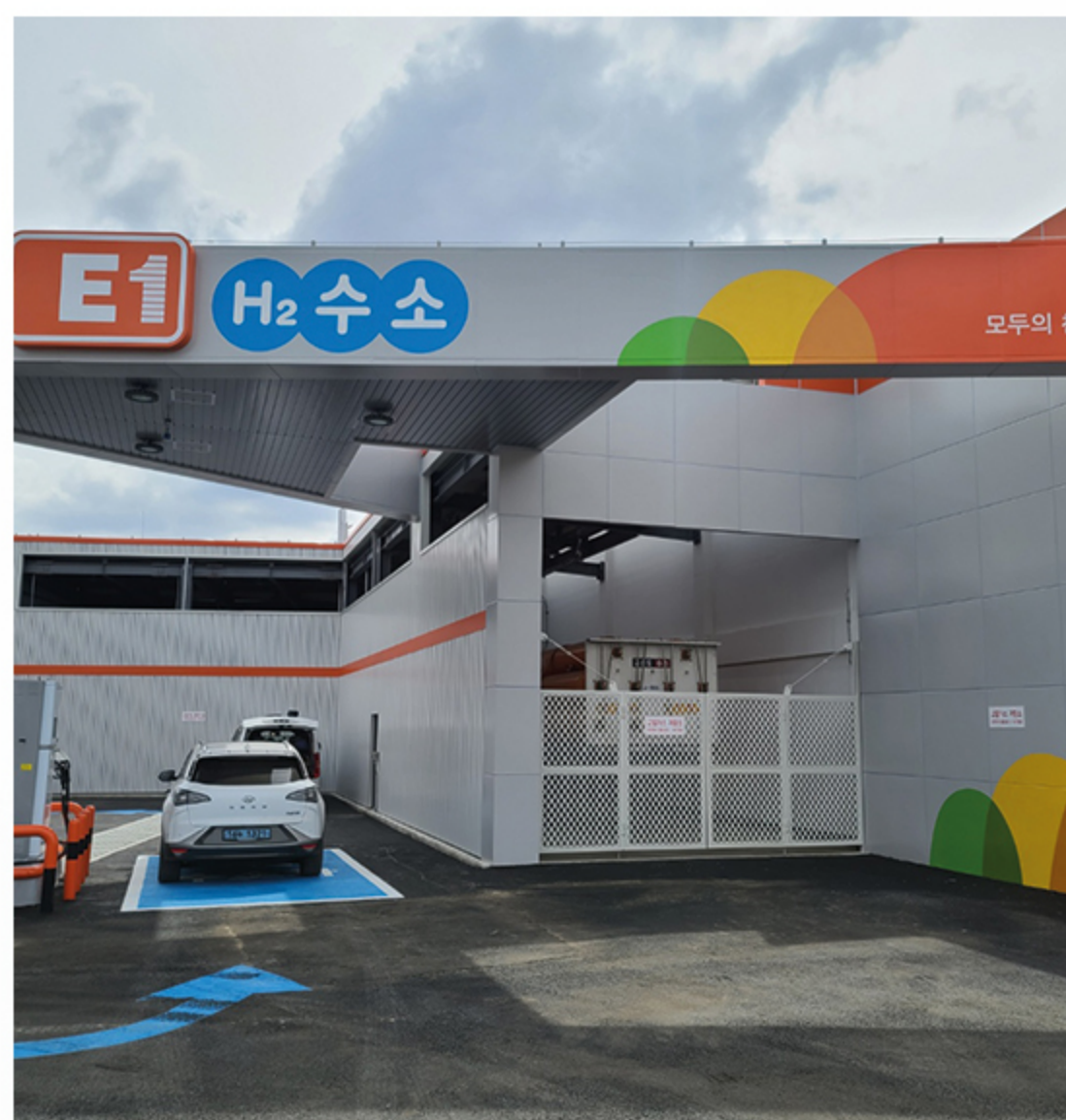
Seoul Ogok Fueling Station
