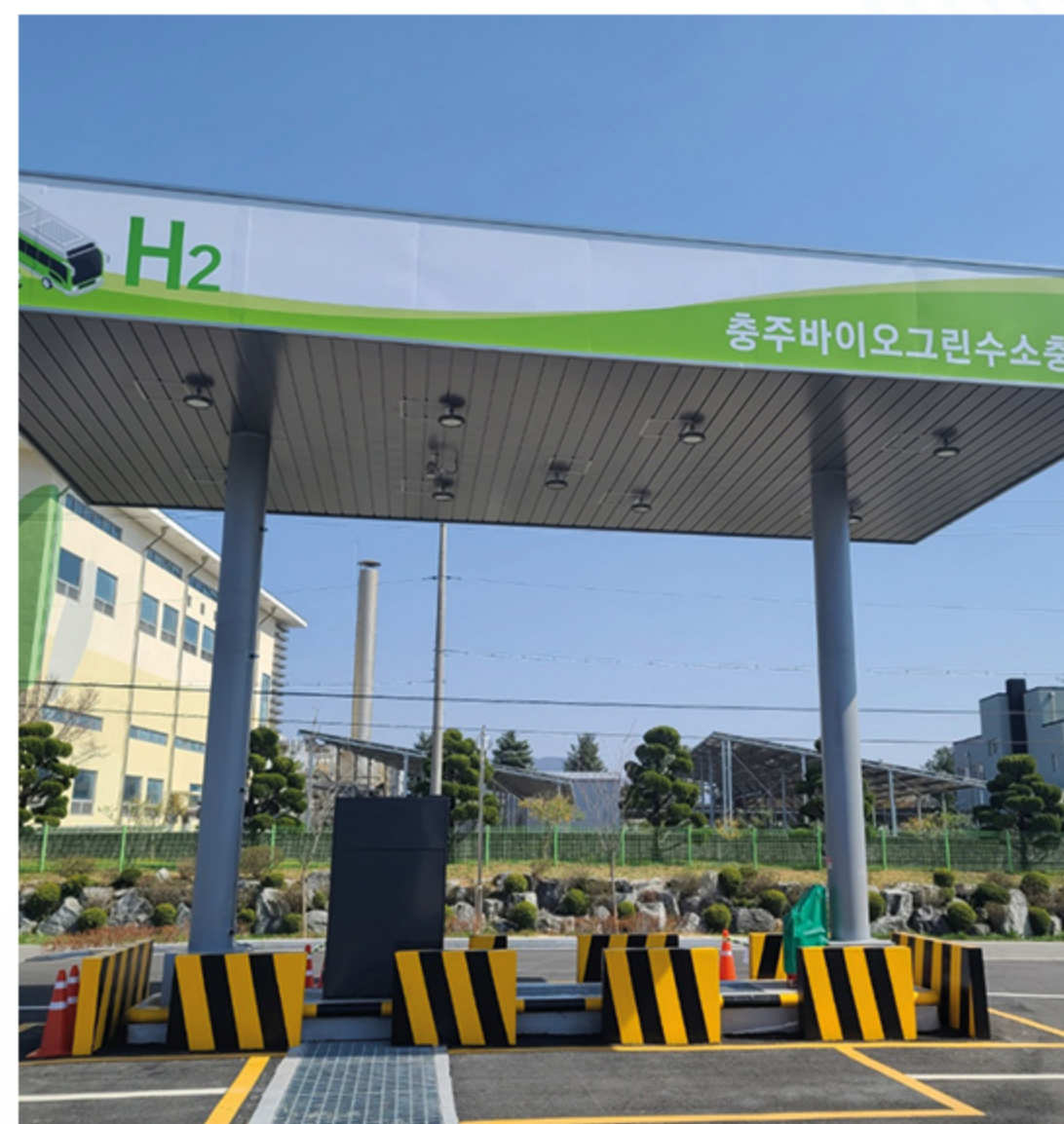
Chungju Bio Fueling Station
