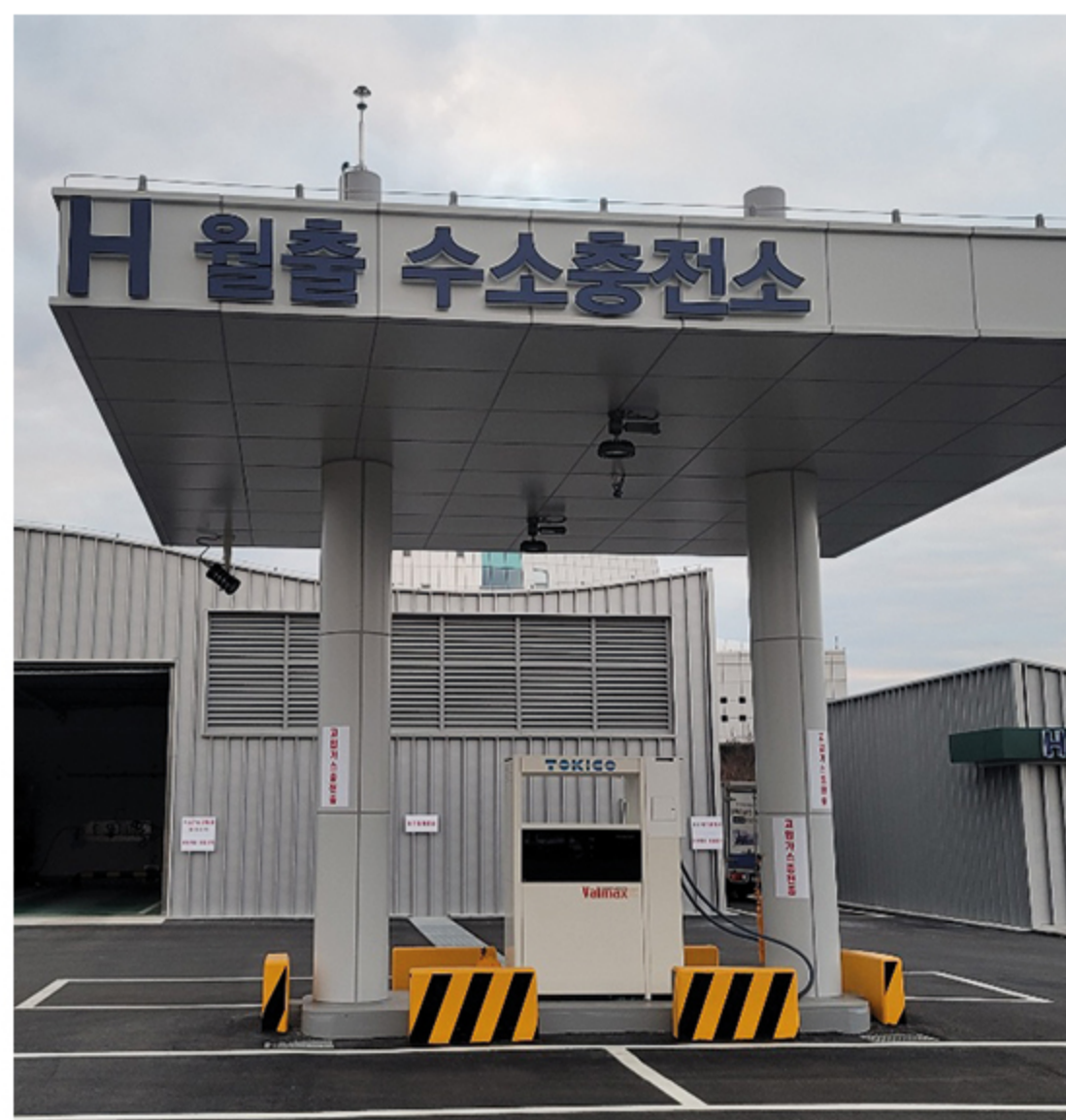
Gwangju Wolchul Fueling Station
