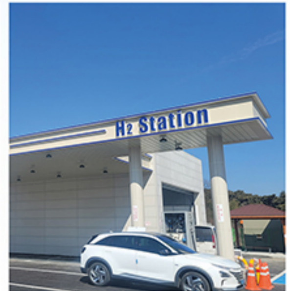
Jeonju Samcheon Charging Station
