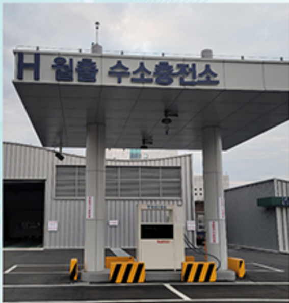
Gwangju Wolchul Charging Station
