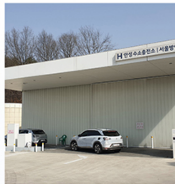
Anseong Service Area Charging Station
