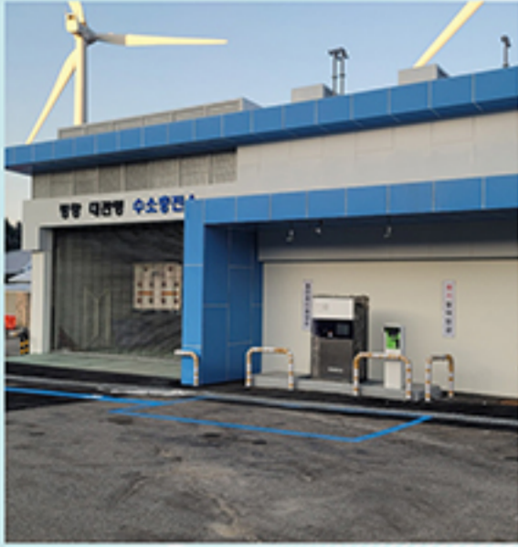
Daegwanryeong Charging Station
