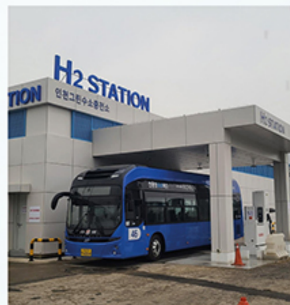
Incheon Jung-gu Charging Station
