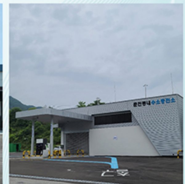
Chuncheon Charging Station
