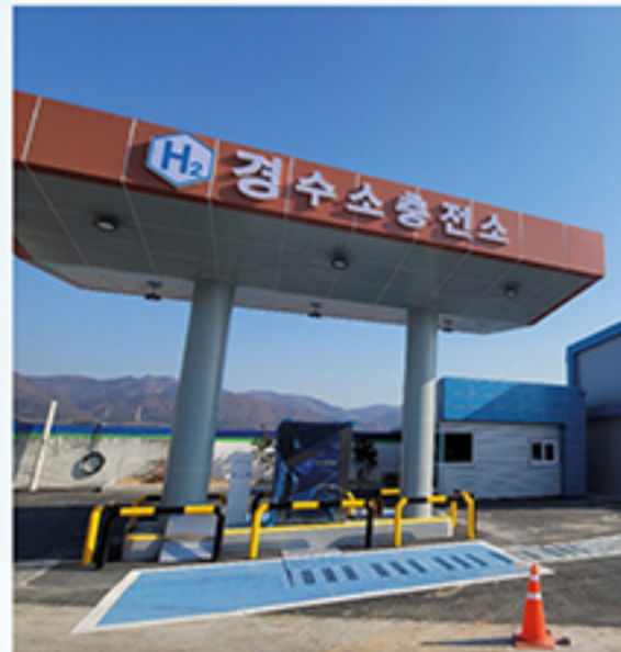
Ulsan Changpyeong Charging Station
