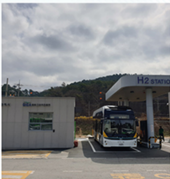
Gwangju Greencar Charging Station
