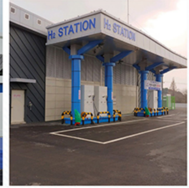
Seosan Charging Station
