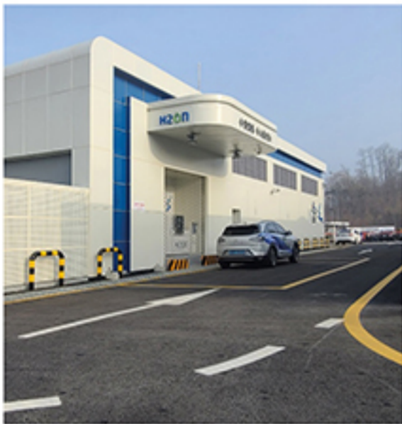
Suwon Gwanggyo Service Area Charging Station
