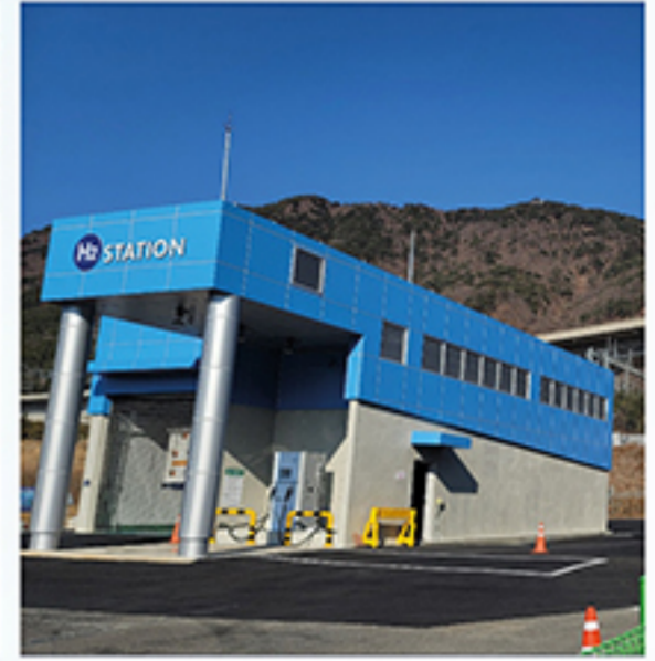
Changwon Sarim Charging Station
