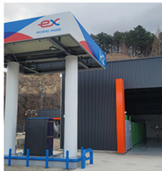
Deogyusan Service Area Charging Station
