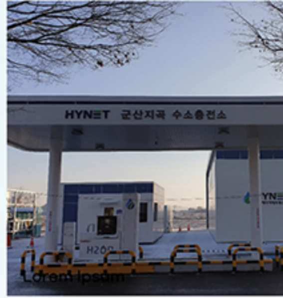
Gunsan Jigok Charging Station
