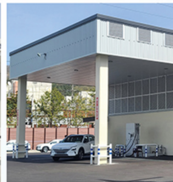
Ulsan Hyundai Motors Charging Station
