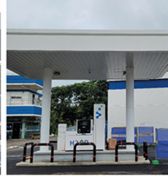
Dangjin Charging Station
