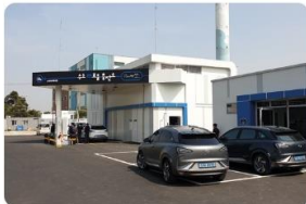
Ansan Fueling Station
