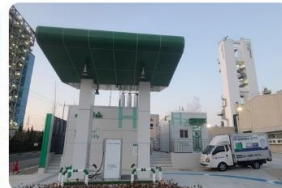
Ulsan APK Fueling Station
