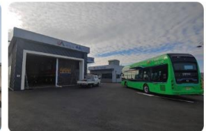
Seosan Fueling Station
